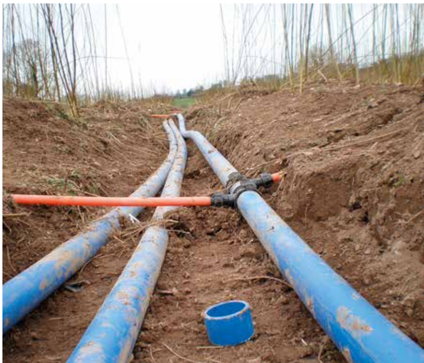
Feed and irrigation pipe construction
