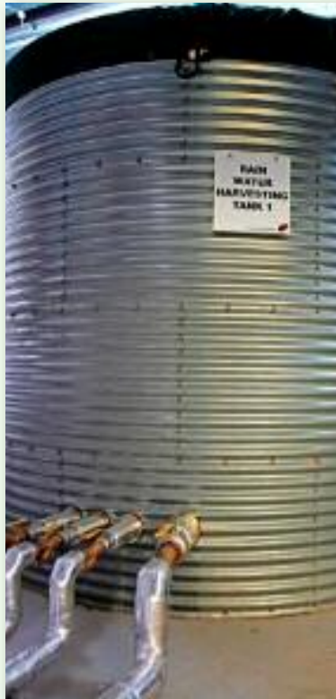
30,000 litre storage tank holding rain harvested water to feed the plate cooler in the new dairy unit at CAFRE, Greenmount.
