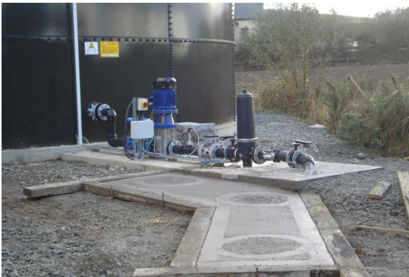
Construction work on high-lift pump at Bridgend WWTW
