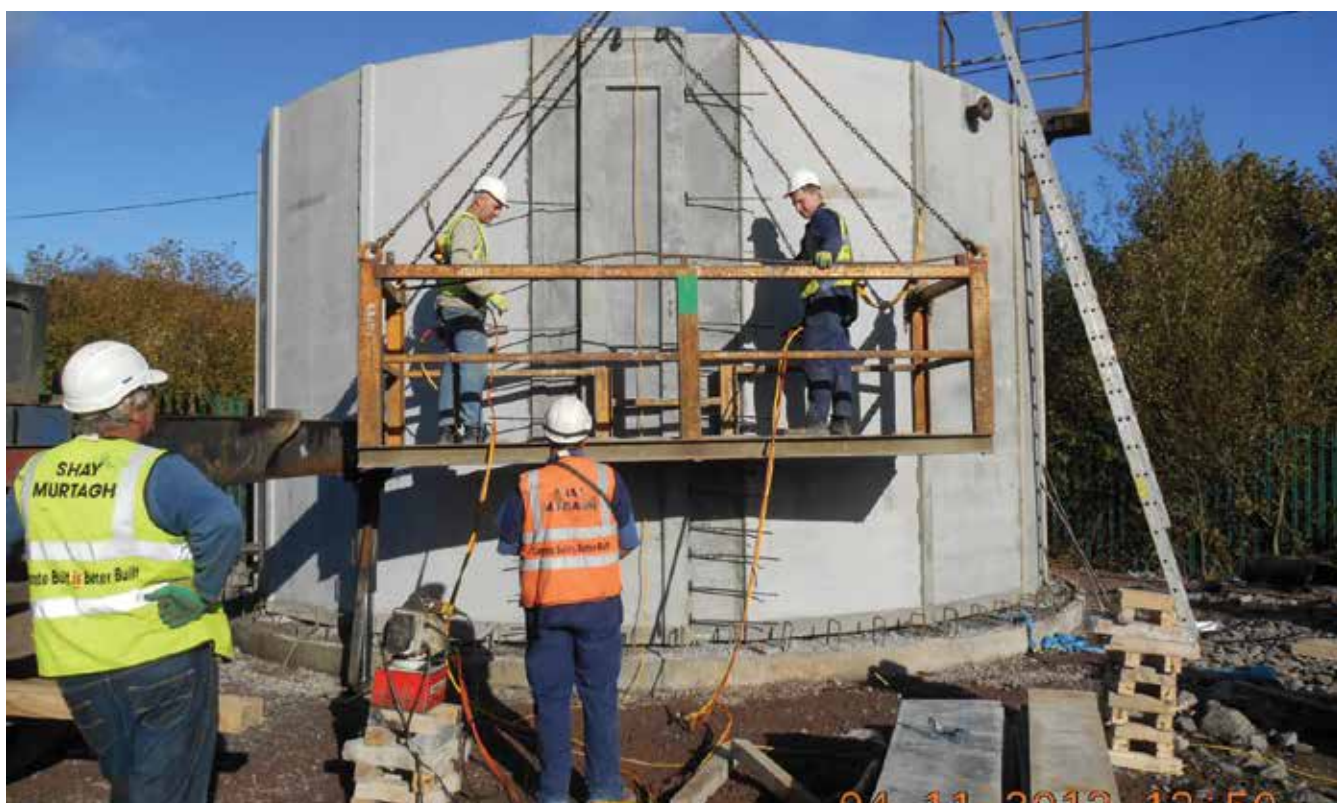
Effluent storage tank at Clontibret WWTWs under construction
