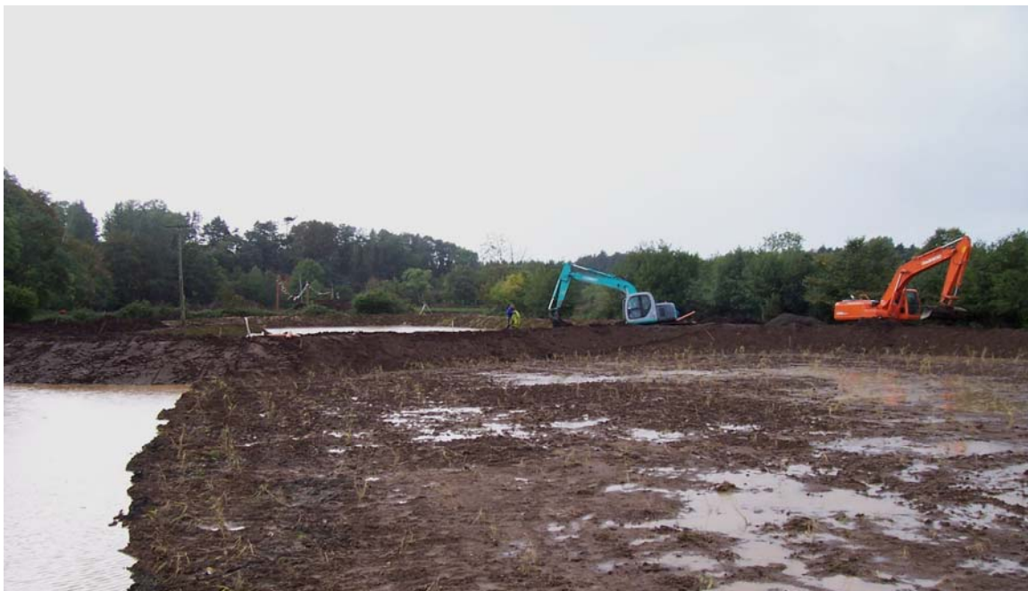
Figure 7 Phragmites australis (Common reed) planted in Pond 1. The excavators in the background were completing bank formation and levelling topsoil
